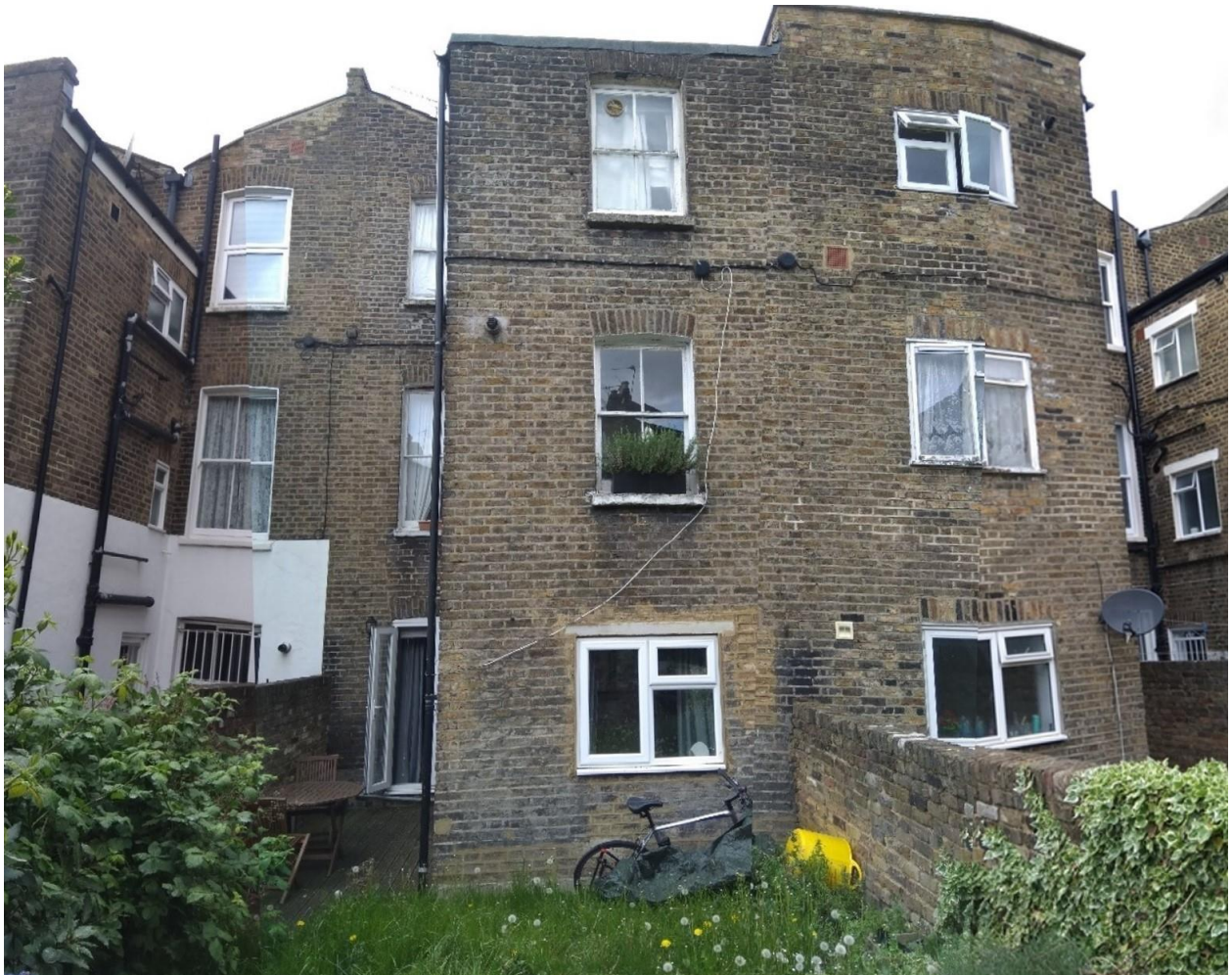
Rear elevation of nos. 53 (left), 55 (centre) and 57 (right) Portnall Road.
