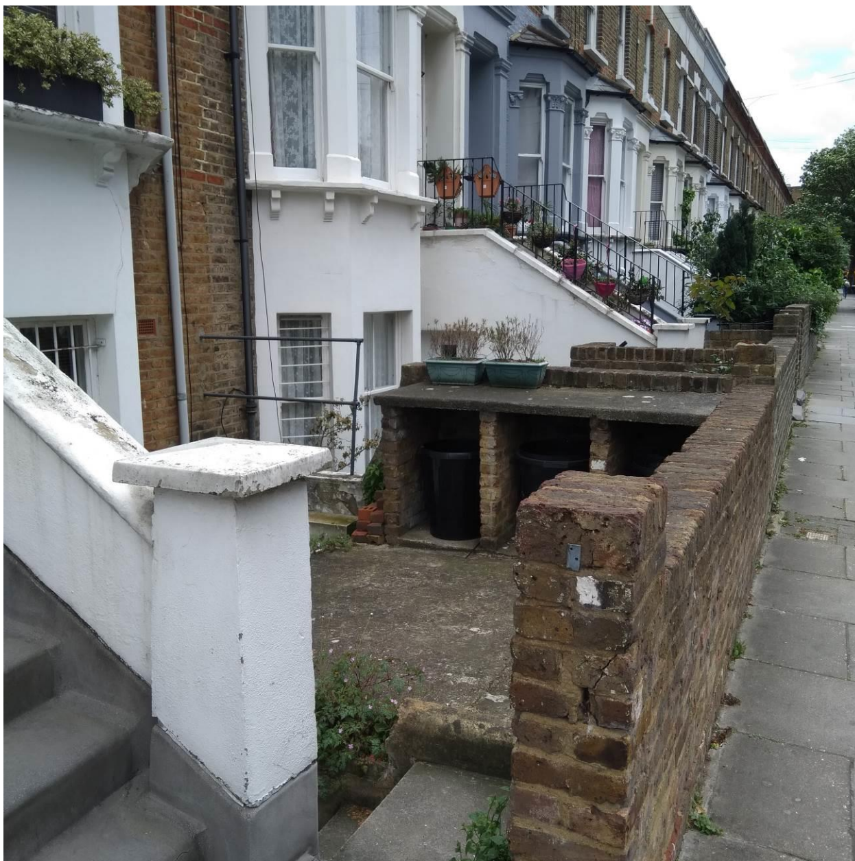
Existing bin store and front lightwell area of 55 Portnall Road.
