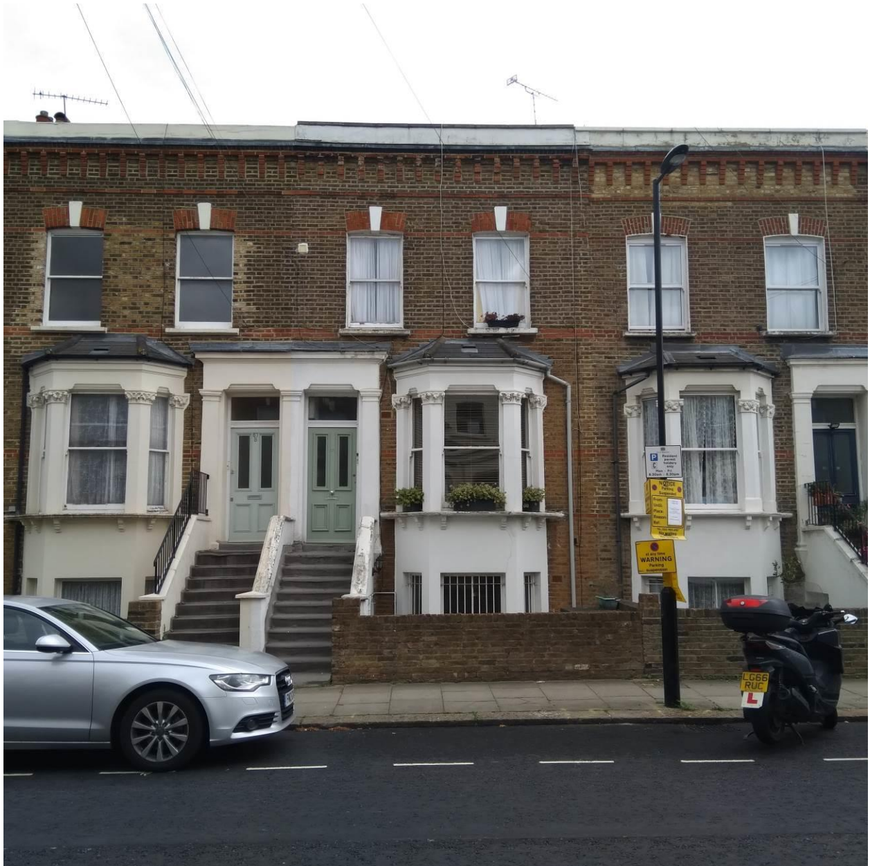
Front elevation of nos. 57 (left), 55 (centre) and 53 (right) Portnall Road.
