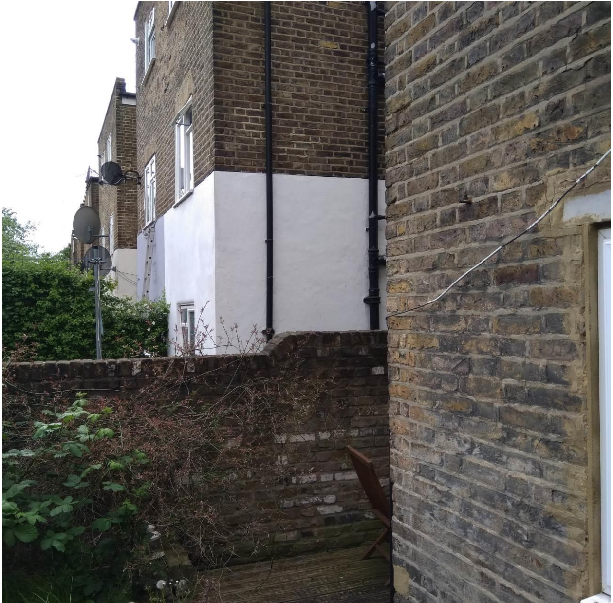
View south from the rear garden of 55 Portnall Road.
